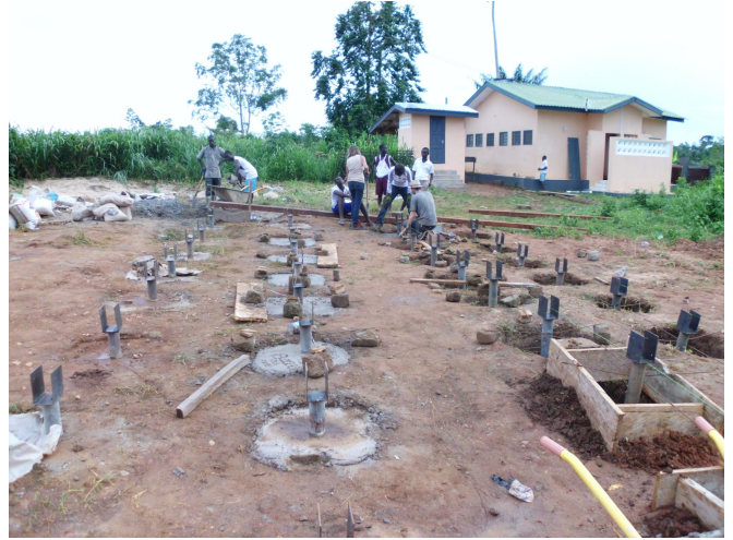
Foundation of Solar plant being laid
