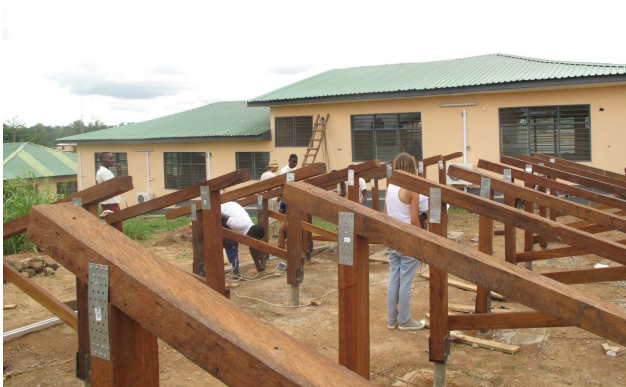
Hard wood instead of Metal Scaffold
